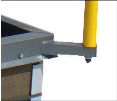
Rail Supports are Welded to Curb
