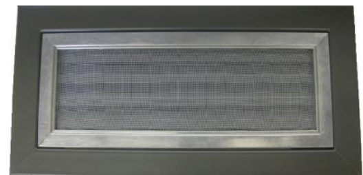
18 x 14 mesh insect screen installed
