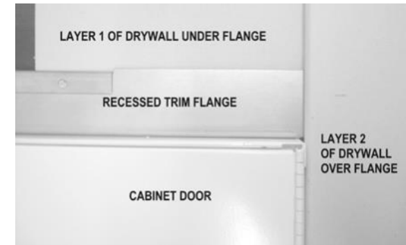
DRYWALL INSTALLATION EXAMPLE
