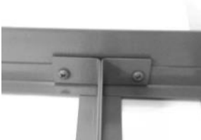
View of Removable Mullion from Underside of Access Panel
