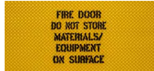
Painted Lettering: Door panel painted in optional yellow with "FIRE DOOR DO NOT STORE MATERIALS/EQUIPMENT ON SURFACE" in black lettering
