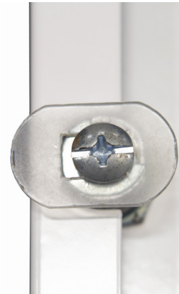
Interior View: Flexible Cam Key Lock
